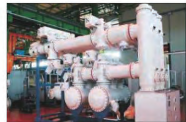
170kV GIS : 3-Ph Enclosed Busbar
