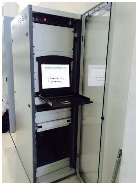
Fig. 8a: Server installation in a Control Room.
