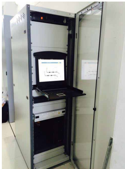
Fig. 8a: Server installation in a Control Room.
