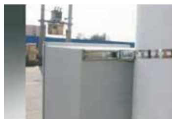
Fixed on the telegraph pole
