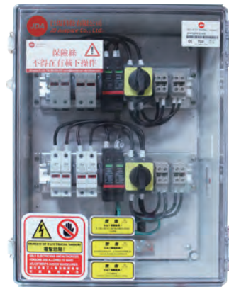
4-circuit-in/4-circuit-out pvBos®
